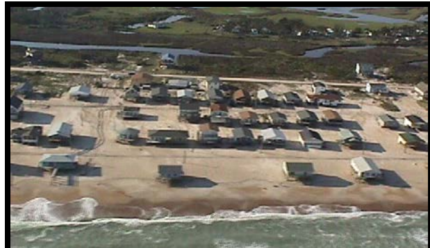
Surf City after Hurricane Floyd
