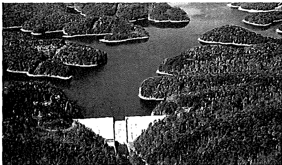
Figure 1. Aerial photo of Philpott Dam.
