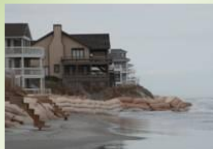
Sandbag revetments along the northern portion of Figure Eight Island
