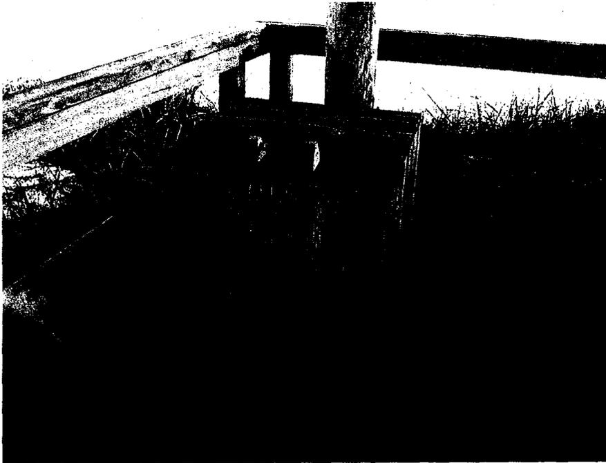
Example of predator proof trash receptacle at Perdido Key State Park. Metal trash can is stored inside. Cover must be tight fitting and made of material heavy enough to stop animals such as raccoons.
