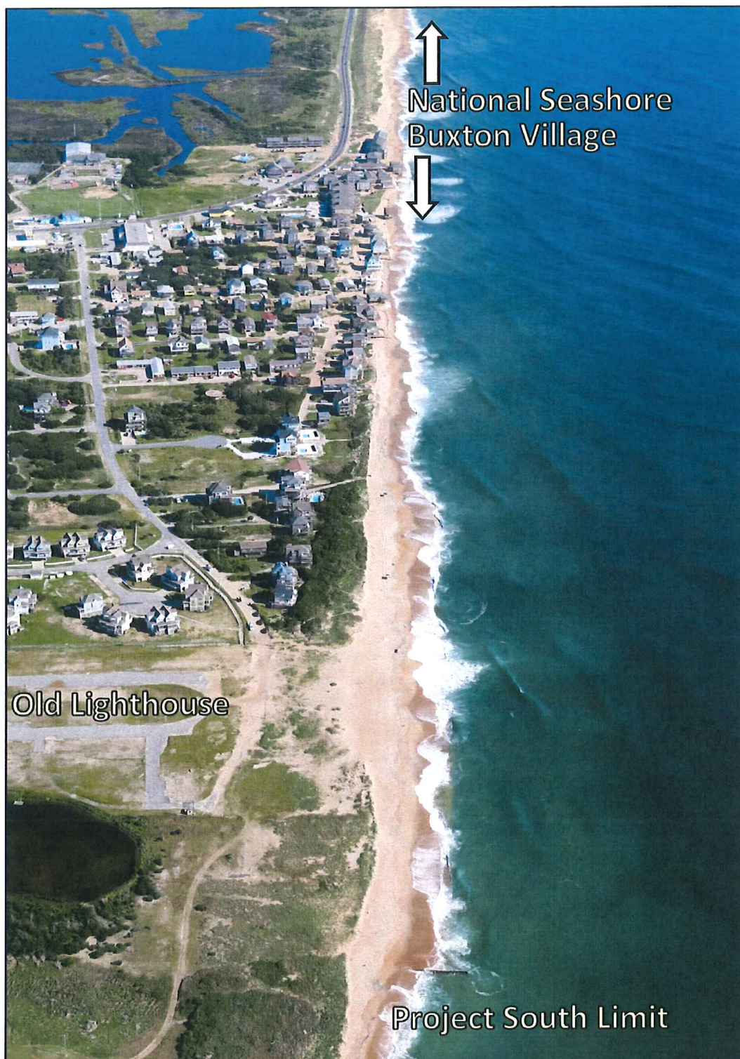
Figure 3 (2 of 2). Aerial image taken by the project team on 11 September 2014 – looking north. The Village of Buxton north limit is located approximately at the end of the northernmost building showing in the photo.
