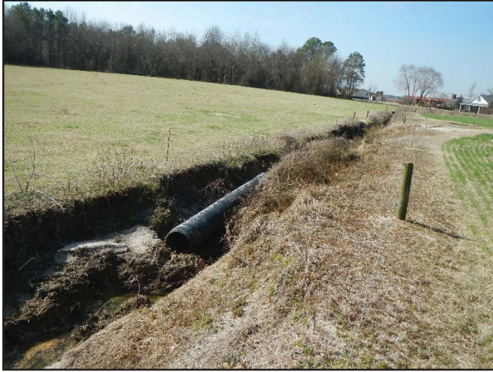
Sadler's Branch, upstream. Restoration Reach
