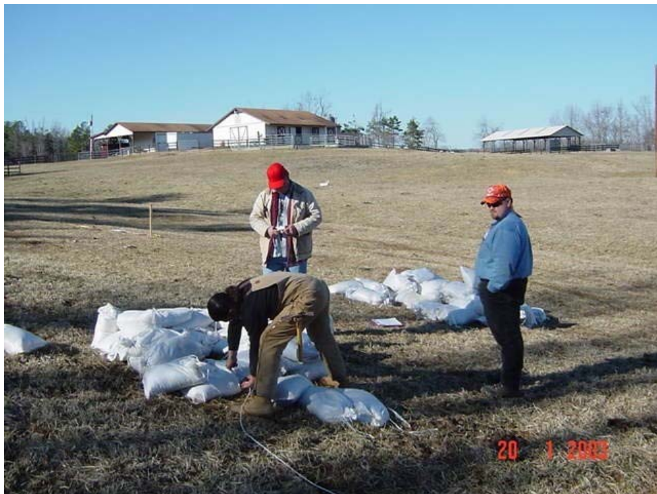
Photo C.12 Demolition Shot Preparation
