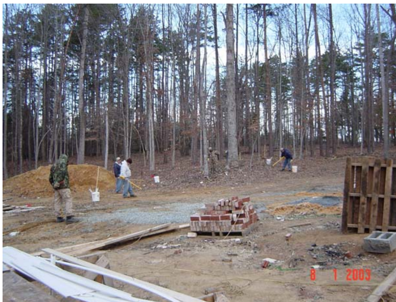
Photo C.2. New House Construction in Lakeview
