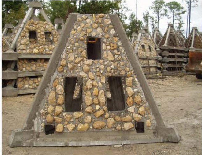
Figure 5. Typical Reef Pyramid design – a cave-like structure, with a 3.65 meter triangular base and a height of 2.44 meters.
