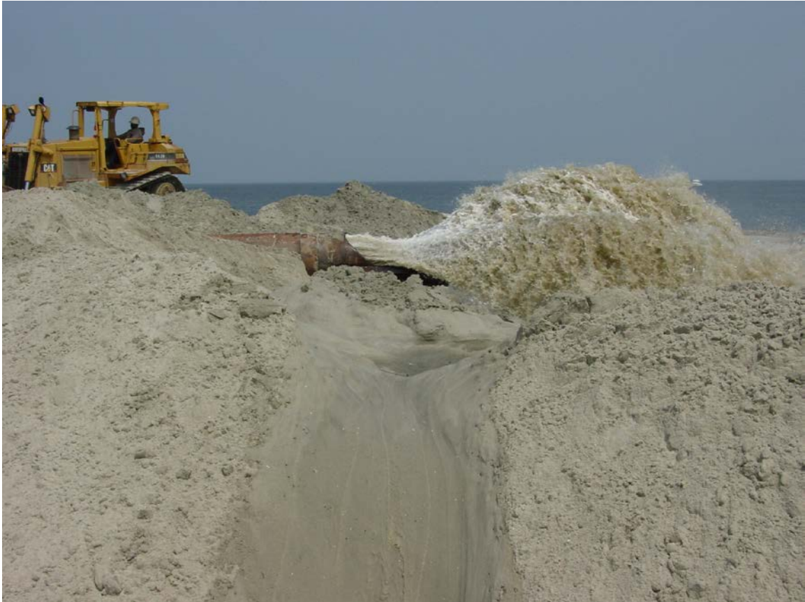
10 11 Figure 5.1. Example of beach fill being constructed (Masonboro Island, NC).
