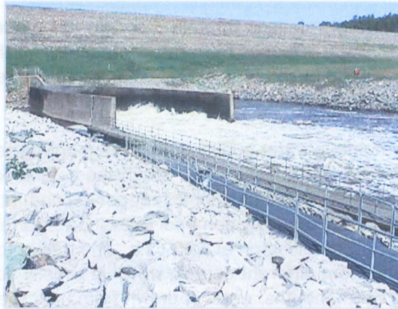
Outlet Works Below Dam
