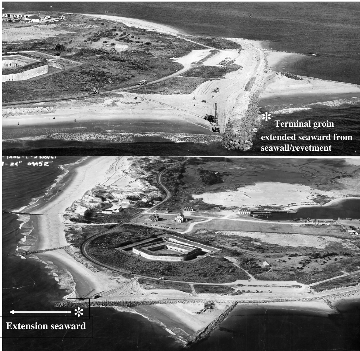
Figure 6. Picture of Fort Macon terminal groin under construction from Nov 1961, and showing all the hard structures placed around the perimeter to try and offset the shoreline erosion.
