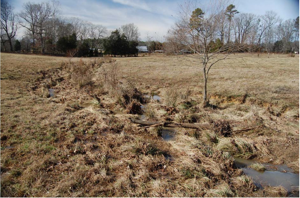
Photo 1: Upper reaches of Motes Creek facing downstream at livestock trampled channel.
