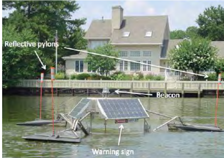
Figure 16 - Visibility and Safety Features of Operating Circulators
