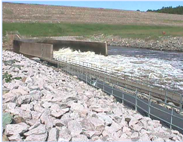
Outlet Works Below Dam
