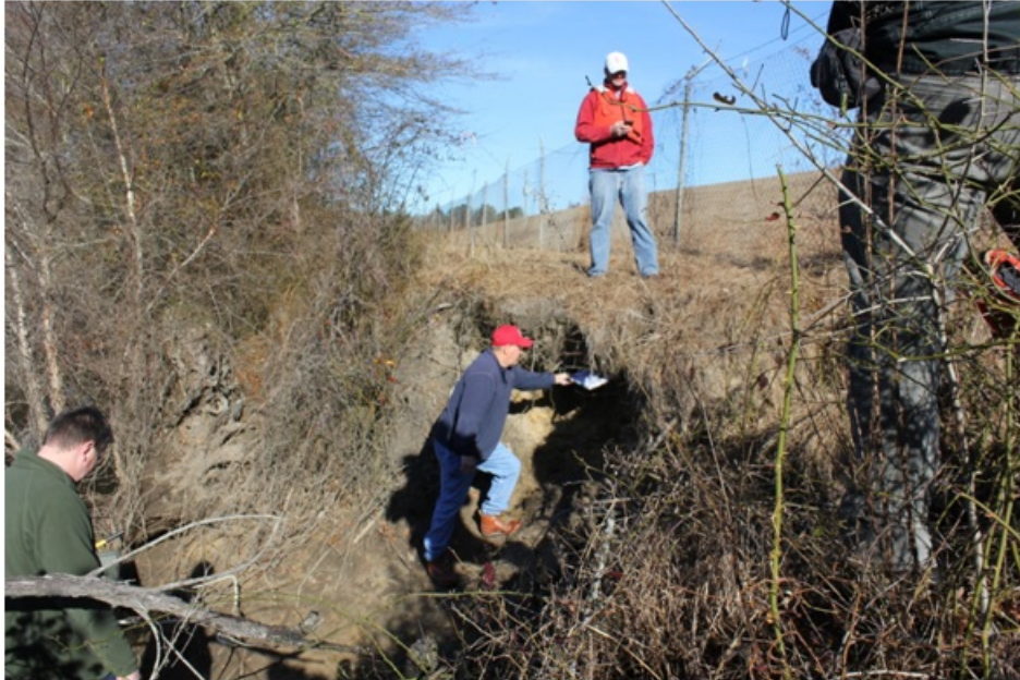
Figure 2.2. Erosion and undercutting at toe of berm.
