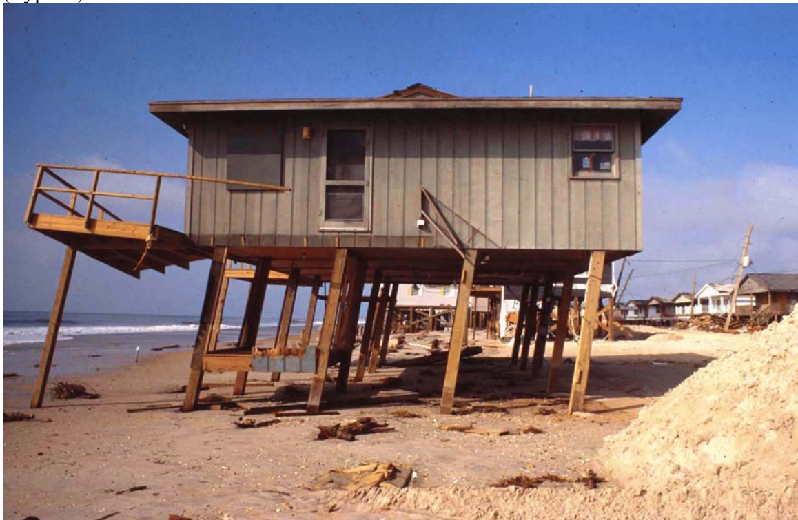
Figure 4: Short piling foundation (Class 1b) near failure on low-elevation shoreline (Type B). Location: Surf City NC after Hurricane Fran.
