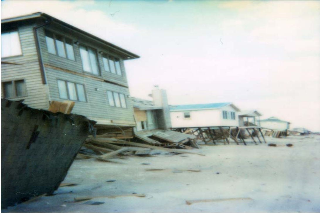
Figure B-11 - Hurricane and storm damage after Hurricane Fran 1996
