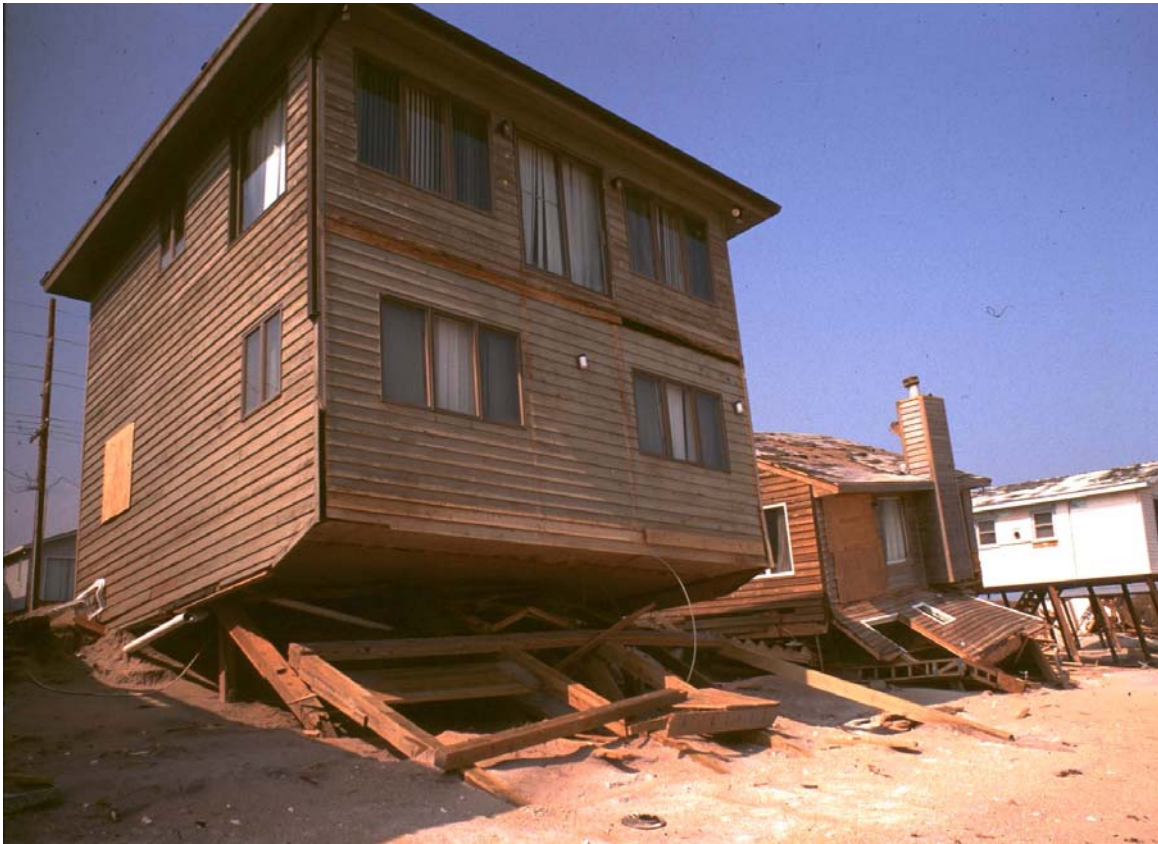
Figure 3: Short piling foundation failures (Class 1b) on high-elevation shoreline (Type A). Location: Kure Beach NC after Hurricane Fran.
