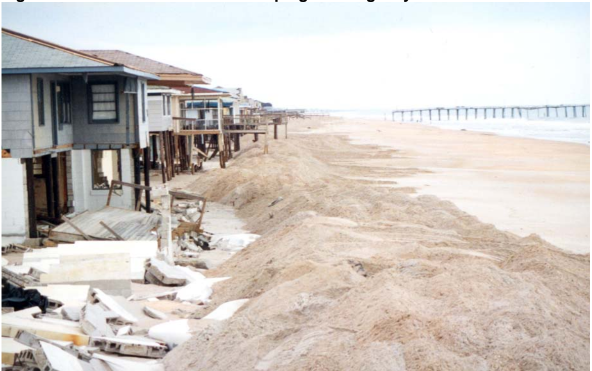
Figure B-4 - Beach scraping following Hurricane Fran
