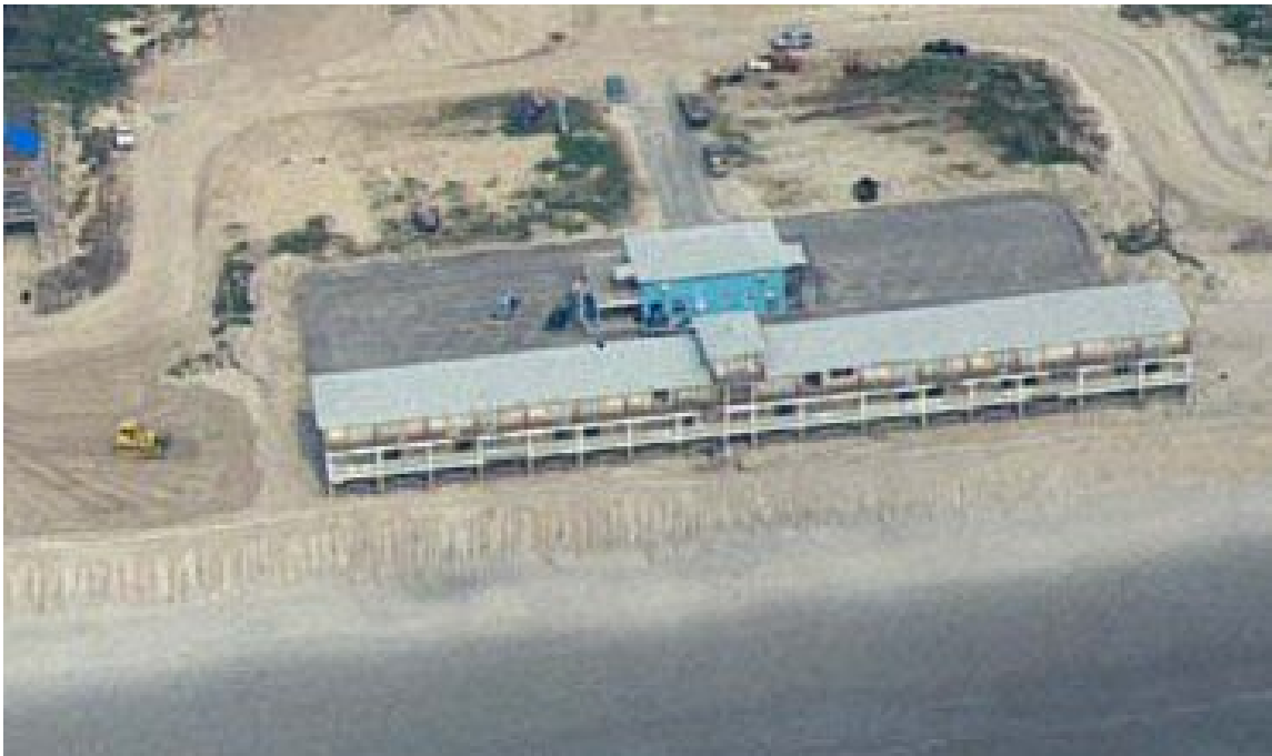
Figure B- 7 - Ocean front hotel at Topsail Beach aerial view following Hurricane Bonnie 1998. Note dune scraping following emergency.
