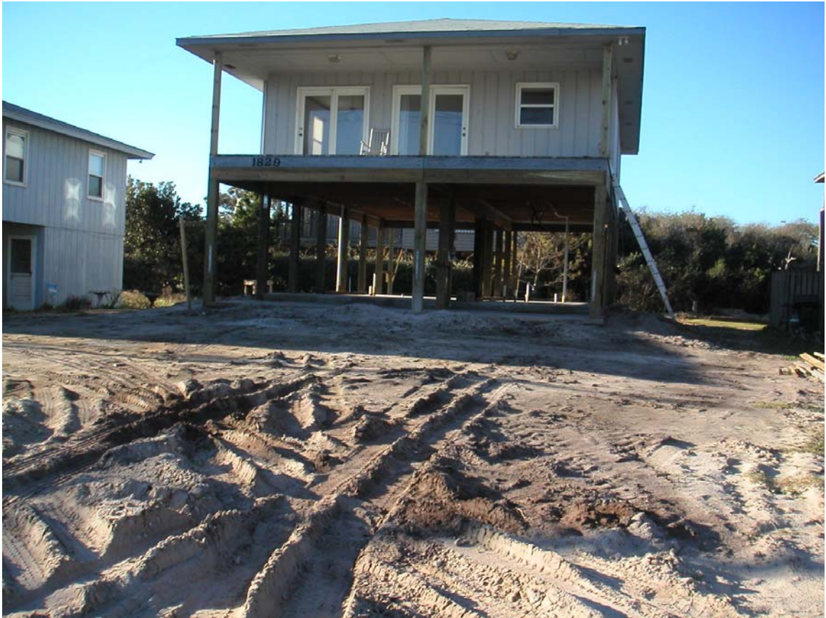
Figure B- 21 Topsail Island home raised on piling foundation 2004.
