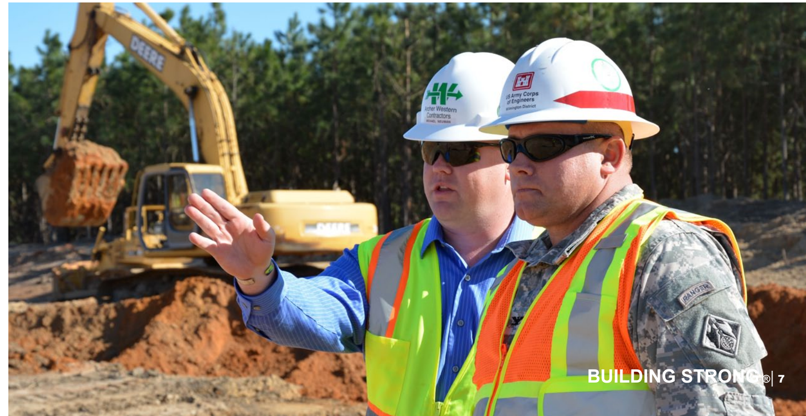
Contractor Michael Neuman (left) discusses areas of the future 3rd Special Forces Group operations facility with Wilmington District Commander Army Col. Steven Baker during the start of construction. The state-of-the-art facility will consolidate the group in one location. (USACE Photo by Jerry Green)
